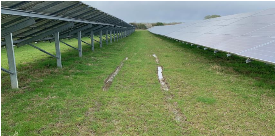
Insert 45: Ruts Caused by Vehicles
