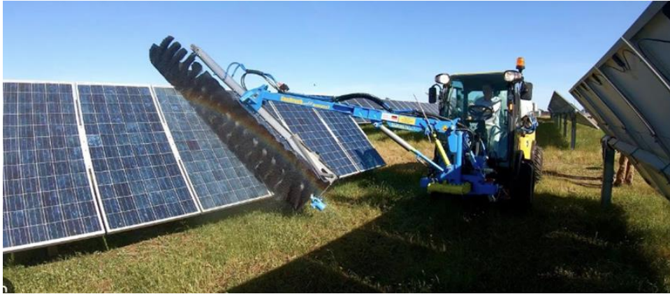
Insert 44: Cleaning of Solar Arrays
